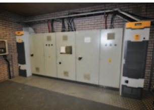
Above: Parker's AC890PX high power, large scale, modular systems drives Right: Siemens' motor drive technology
